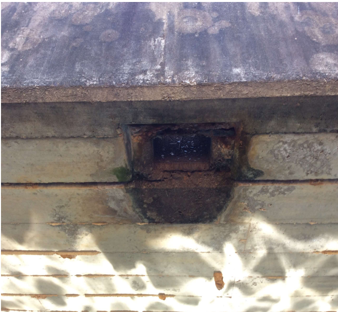
PHOTO 1 Description Spalling with exposed reinforcing steel around both deck drains in Span 2. Exposed reinforcing steel has active corrosion and layers of rust.
